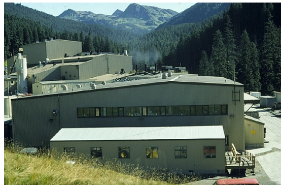
Greens Creek mill as it appeared in 1996. Credit: Tom Bundtzen
